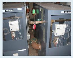
These ALM controllers do not require calibration, they infer boiler temperature settings and are compatible with OTR systems
